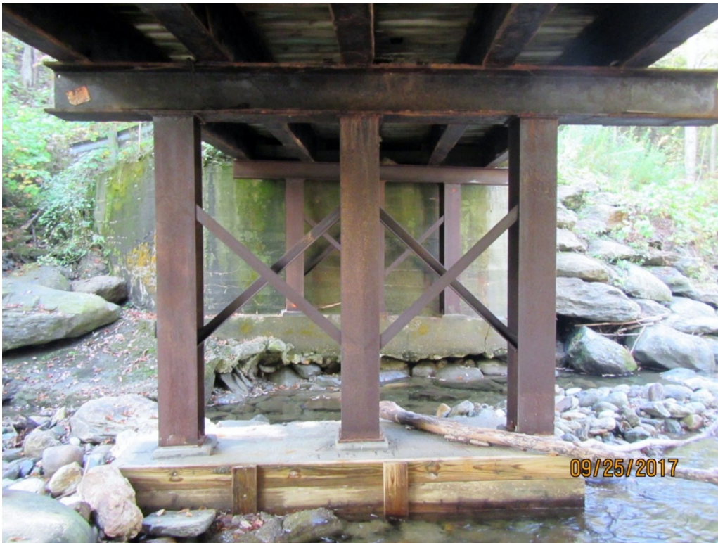
Picture 5: Temporary Mid-Span Support – Note undermining at far abutment
