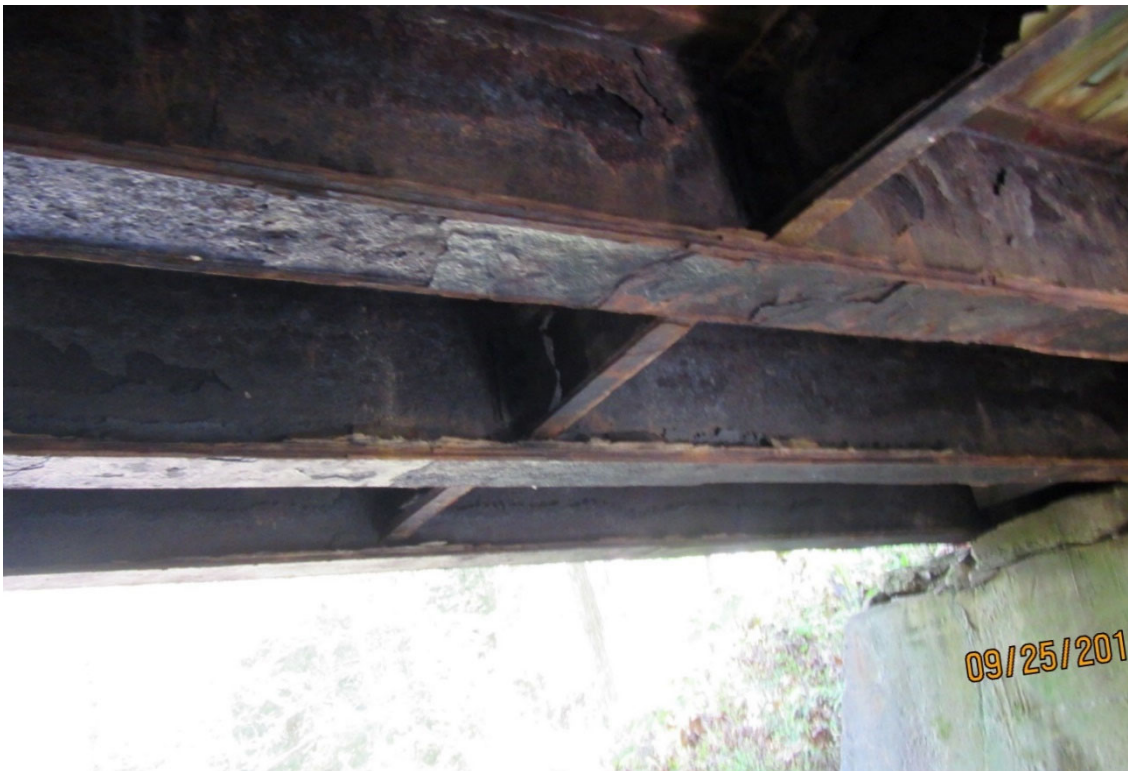
Picture 6: Significant Corrosion of Beams
